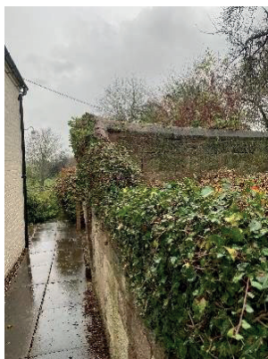
Job to be done
